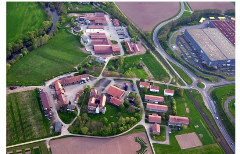
Agricultural test site for grid integration of biogas derived energy (power, heat, gas)
