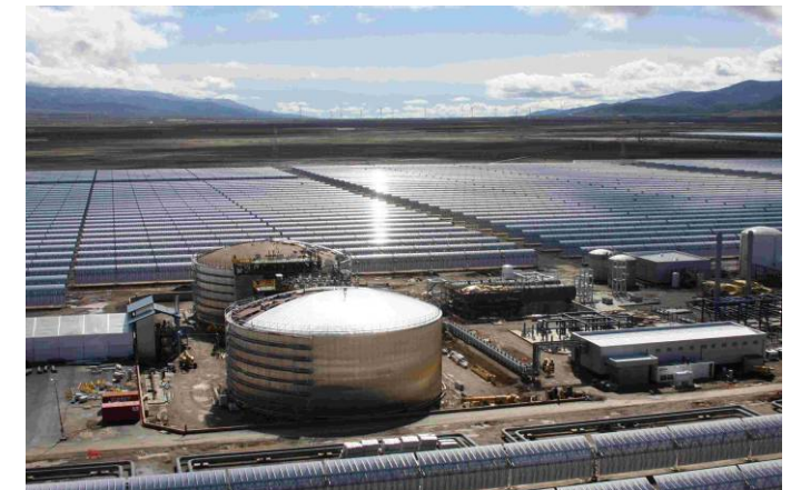
Andasol 50 MW power plant in Spain (Copyright: Solar Millennium AG)
