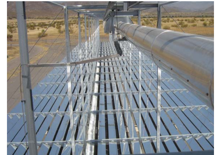
Primary mirror field of Linear Fresnel Collector (FRESEMO, Almeria, Spain)
