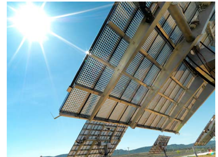
CPV Tracker using FLATCON® modules (source: Concentrix Solar)
