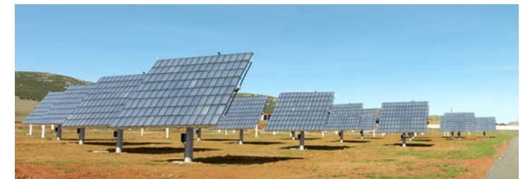
CPV power plant in Puertollano (Spain) equipped with the Tracking Inverter and using the MPPTm (source: Concentrix Solar)
