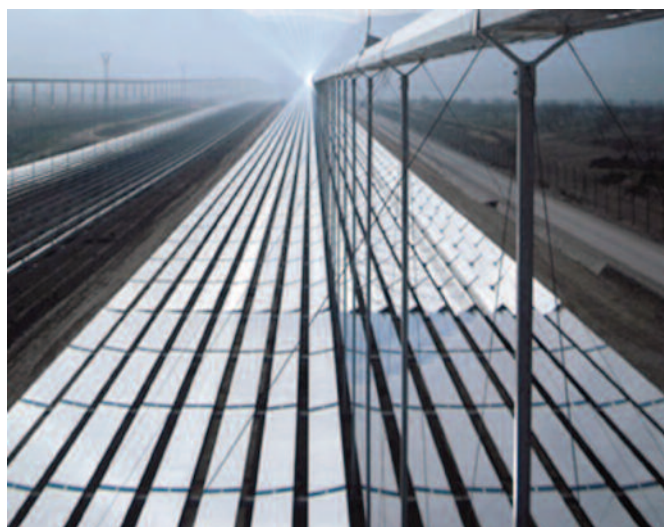
Figure 3 Collector array of the first solar thermal power plant with direct solar evaporation near Murcia (Image: Novatec-Biosol)
