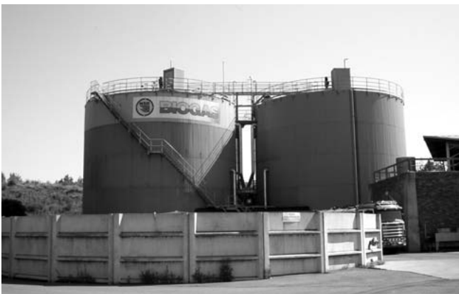
Picture 2: Mesophilic digesters in the city of Helsingborg for co-digestion of manure and animal waste
