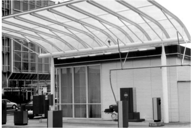
Figure 4 Public LH 2 filling station at airport Munich
