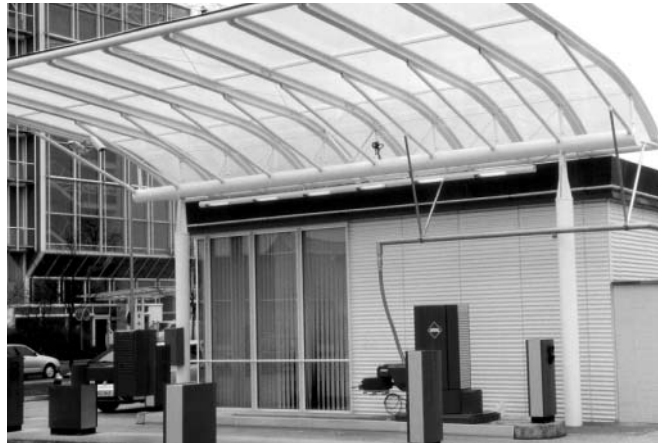
Figure 4 Public LH 2 filling station at airport Munich
