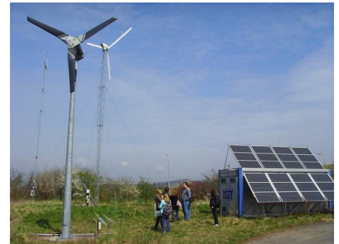
Small wind turbines at Fraunhofer IWES test site near Kassel
