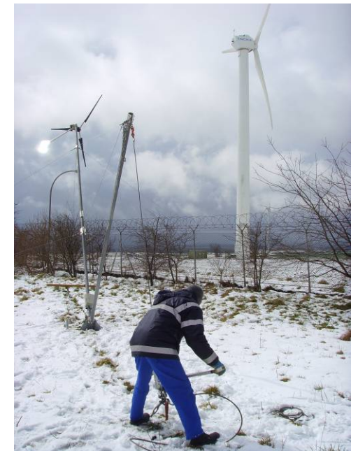
A small wind turbine at Fraunhofer IWES test site is lowered to the ground for maintenance
